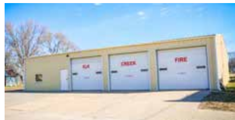
The community of Elk Creek completed a new fire hall and community building last year, made possible with support from the Elk Creek Community Fund.
